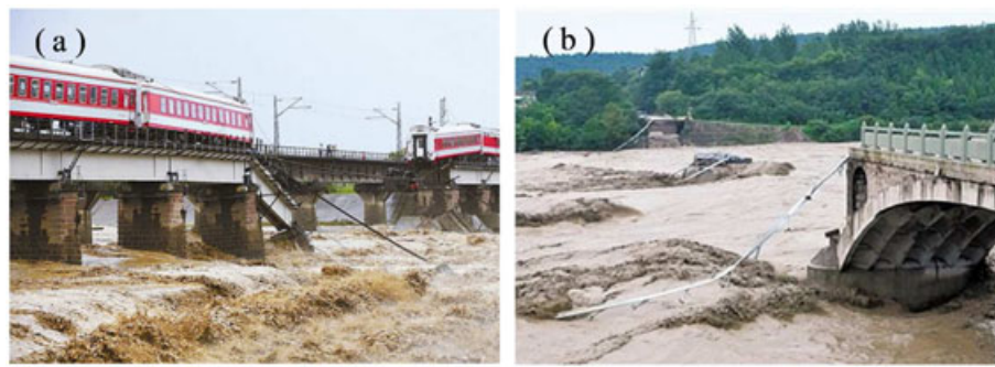
FIGURE 1 Scour-induced bridge collapses. (a) Shi-Ting-Jiang Bridge failed on August 19, 2010 [8] ; (b) Pan-Jiang Bridge failed on March 9, 2013. [9] Both bridges were in Sichuan province, China
